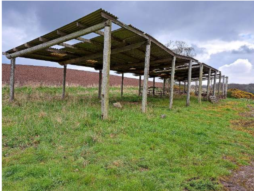
Image 8.3 Open shed at Stone Mills
