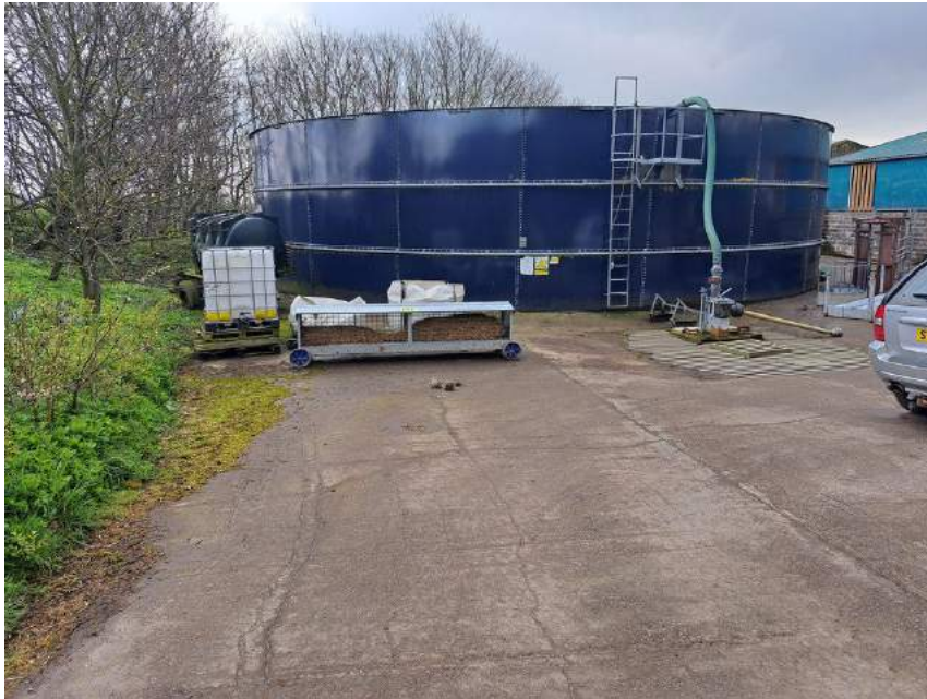
Image 8.5 Slurry tank at Wester Rora (disused)
