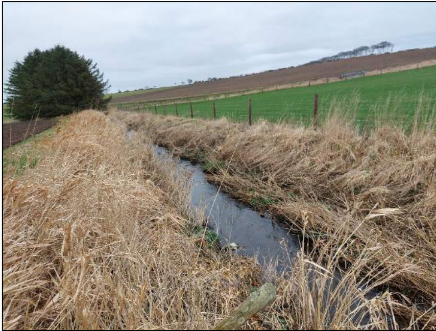
Photo 7.2 - Example of a channelised watercourse visited during the field surveys, located at BNG 400462, 844520
