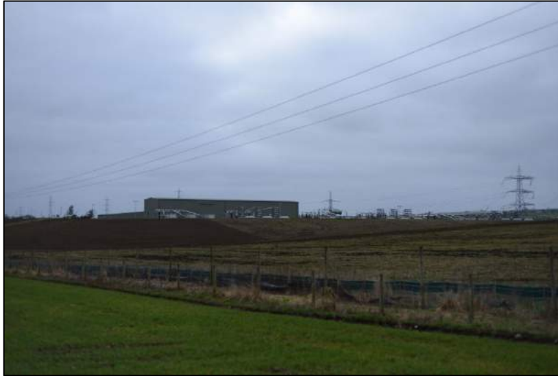
Image 4.7 – The Existing New Deer Substation
