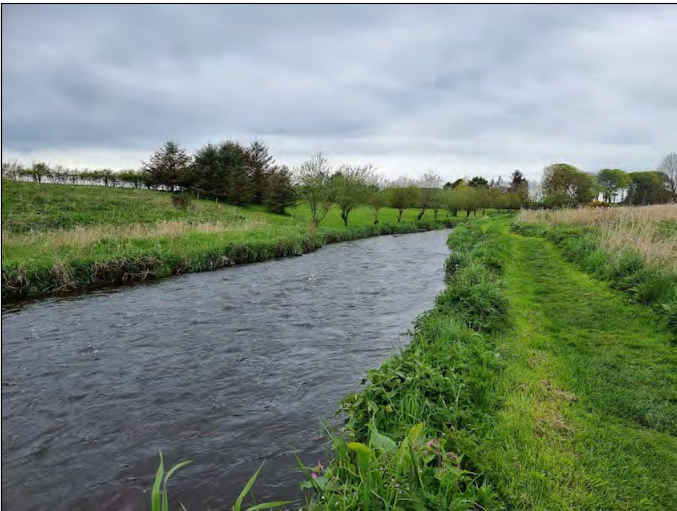
Figure 16. The River Ugie at a proposed trenchless crossing point.
