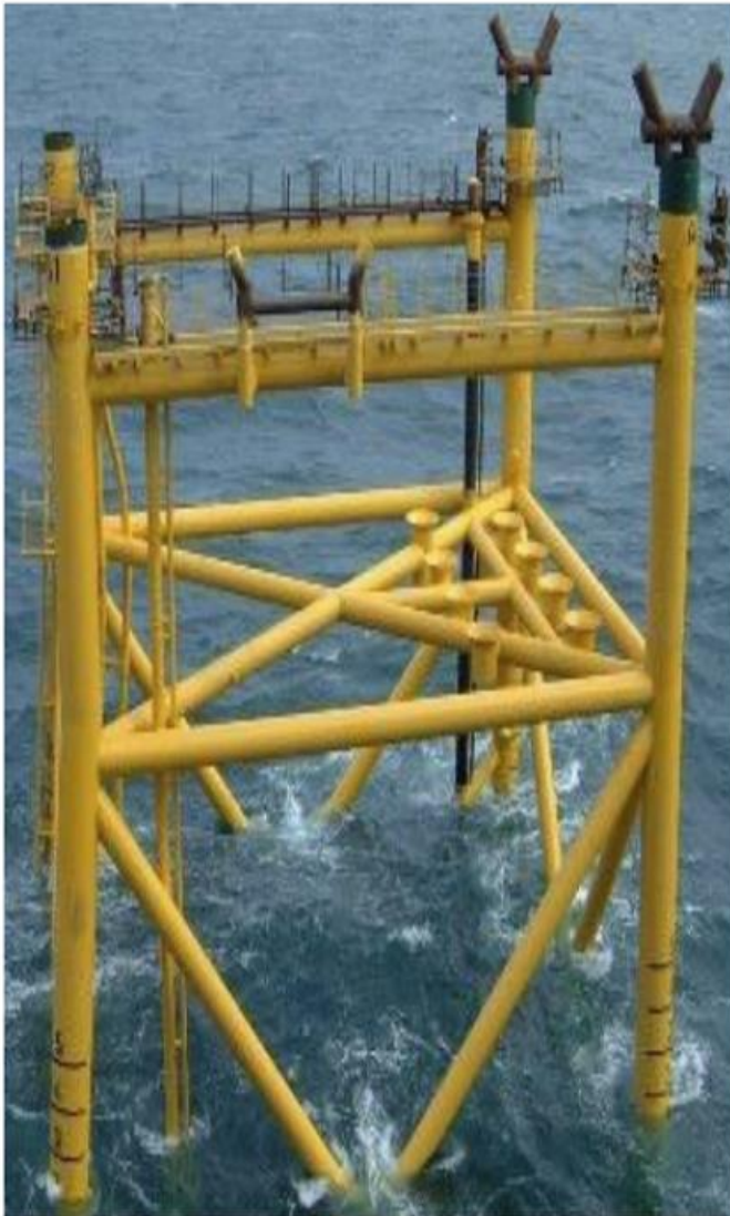
Figure 5.9 A 4-legged Jacket option used for the Goldeneye O&G Field Platform located in North Sea block 14/29, adjacent to block 20/3 where the Offshore Development Area will be located.
