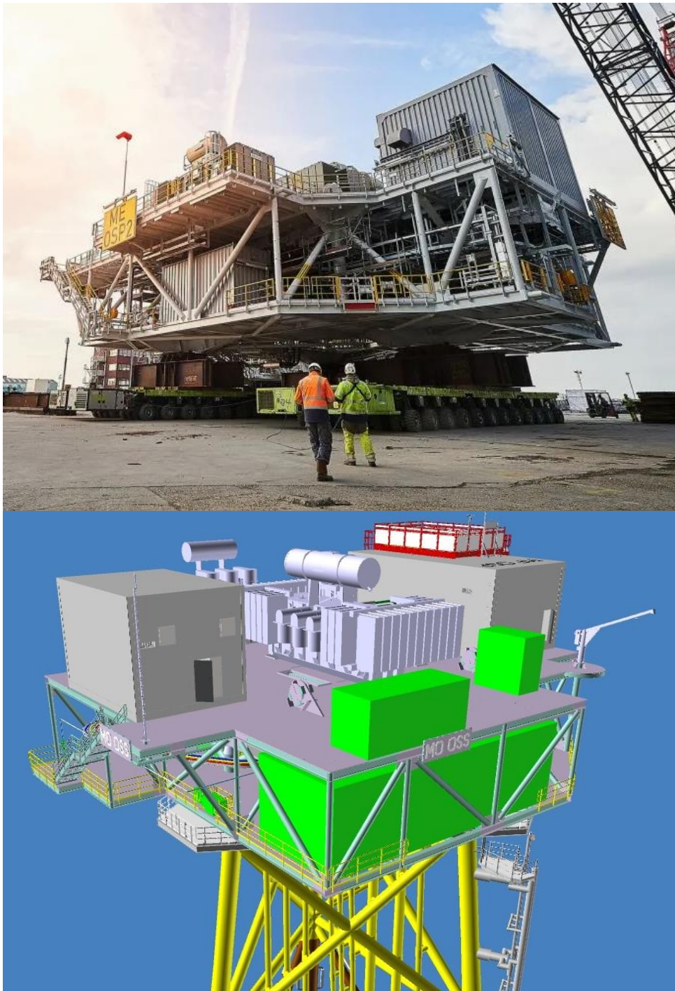
Figure 5.10 Siemens Offshore Transmission Module solution utilised on the Moray East Offshore Windfarm. The Green Volt OSP will be similar. Figures obtained from https://news.siemens.co.uk/news/siemens-wins-order-for-its-largest-offshore-grid-connection-in-the-uk-to-date
