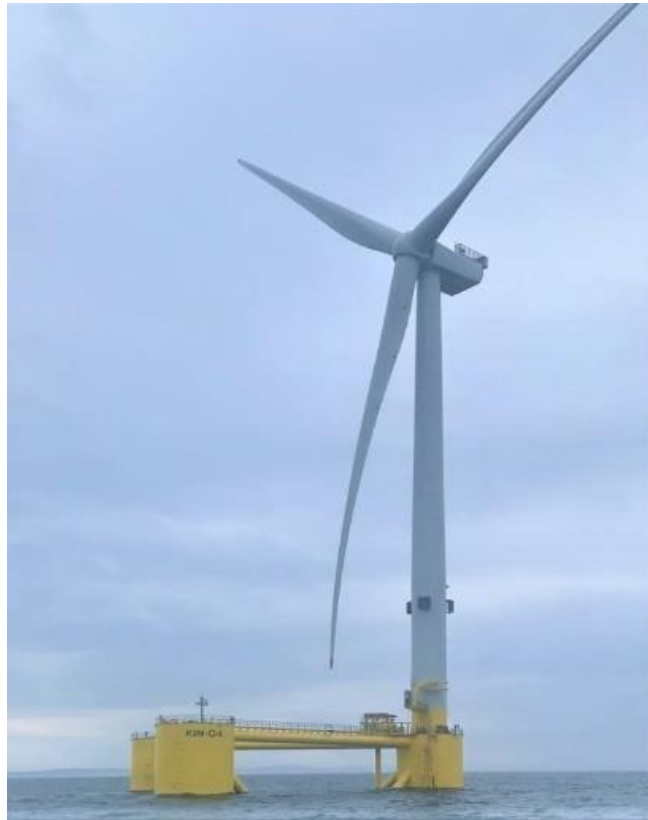
Figure 5.4 A 9.5 MW turbine supported by a semi-submersible substructure as used on the Kincardine floating windfarm
