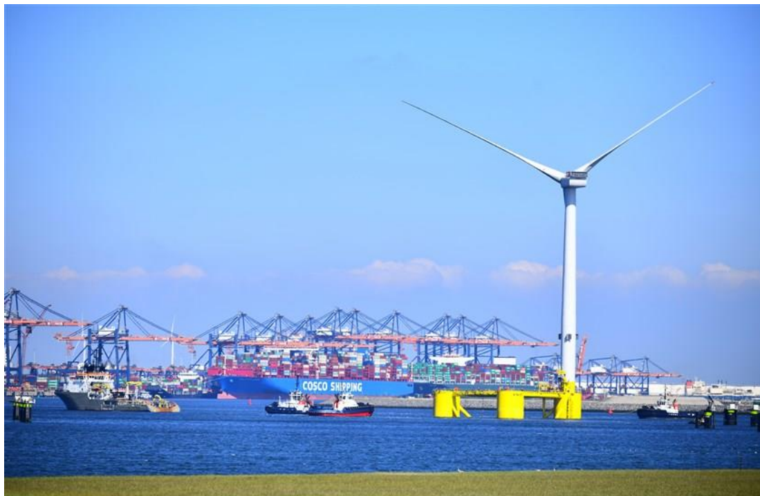
Figure 5.13 Example of WTG assembly onto a semi-submersible platform at quay side. (Source: Kincardine)
