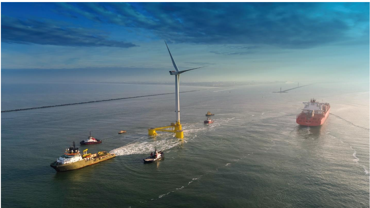
Figure 5.14 Tug vessel towing the Kincardine's integrated WTG and semi-submersible substructure unit out to windfarm site.
