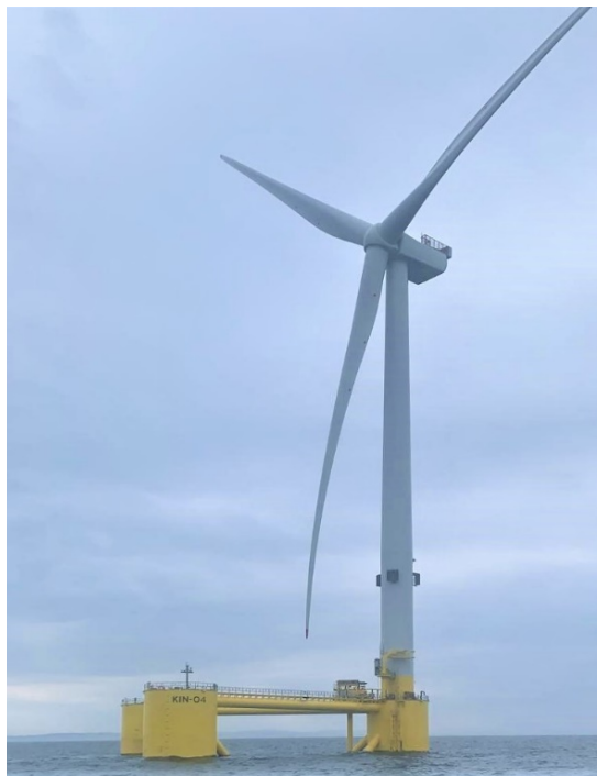
Figure 2.1: Vesta 9.5 MW turbine supported by the PPI Windfloat2 substructure on the Kincardine floating windfarm
