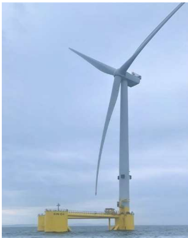
Figure 2.1 Vesta 9.5 MW turbine supported by the Windfloat2 substructure on the Kincardine floating windfarm
