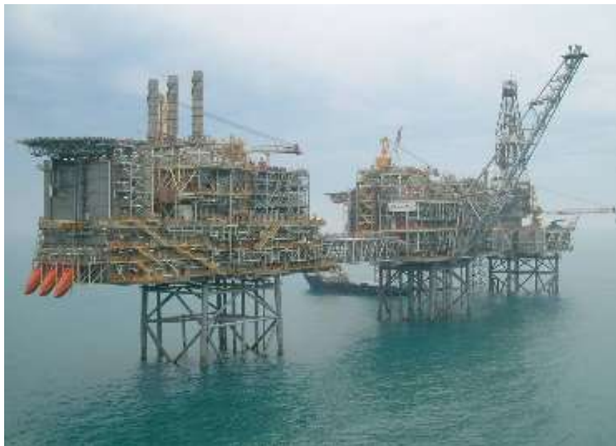
Figure 1.1: Buzzard oil and gas facility, with power generation chimneys visible on the leftmost platform.
